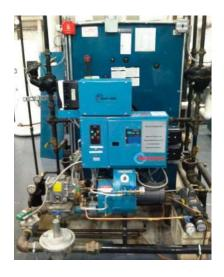
**TEMP-A-TRIM®** saves money on fuel and utilities. Webster Combustion's patented TEMP-A-TRIM air density trim system senses combustion air temperature and automatically varies the fan speed to create a constant air flow mass for combustion. By maintaining optimum fuel/air ratios, TEMP-A-TRIM ensures that the burner is operating at maximum efficiency.
